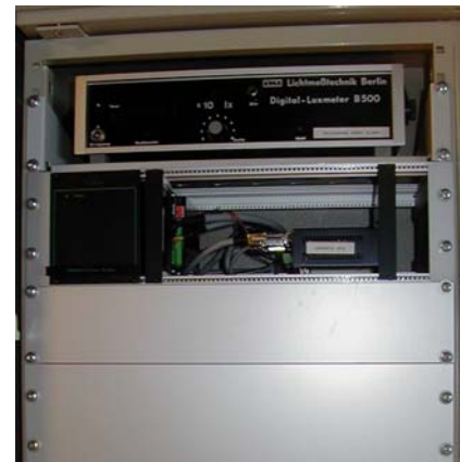
Cabinet with controllers and lux meter
